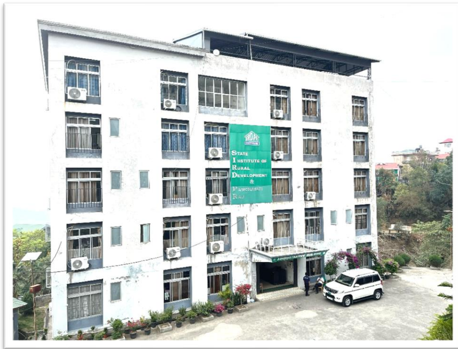
Administrative building of SIRD&PR, Mizoram, Durtlang Leitan
