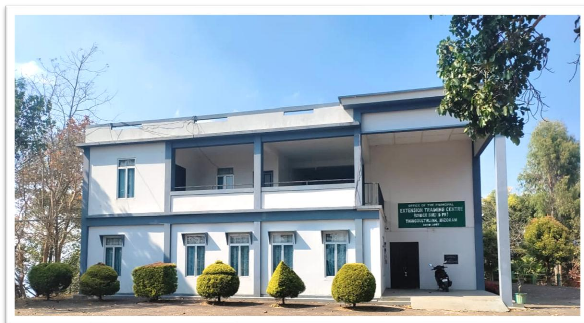
Administrative Building, ETC, Thingsulthliah
