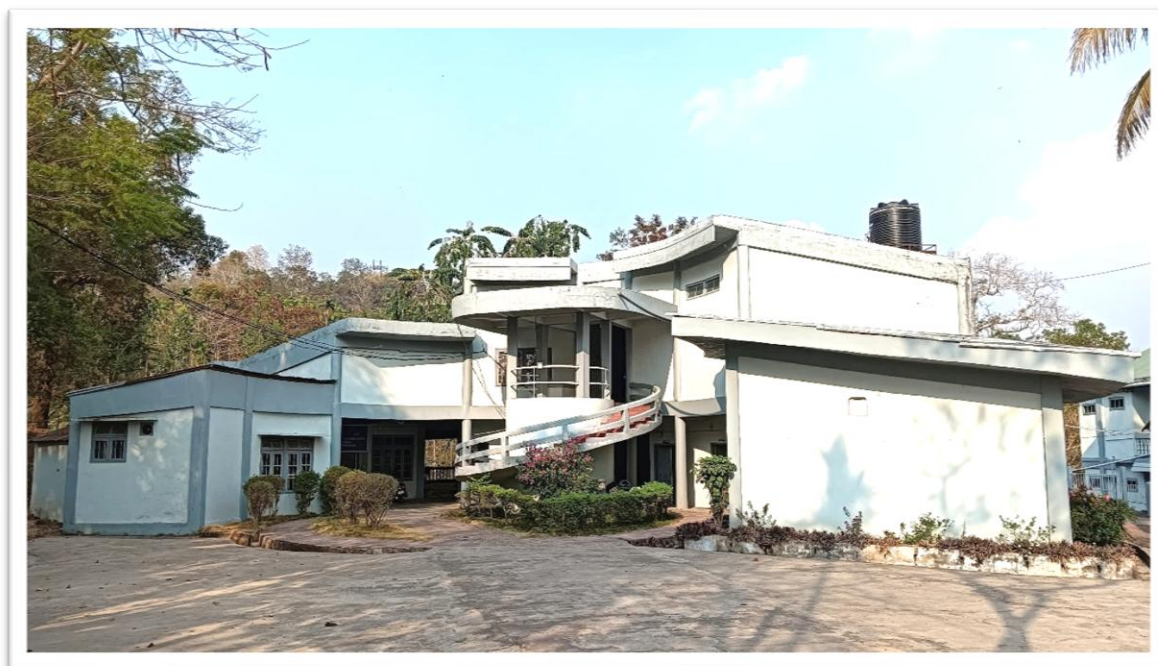
Administrative Building, ETC, Kolasib
