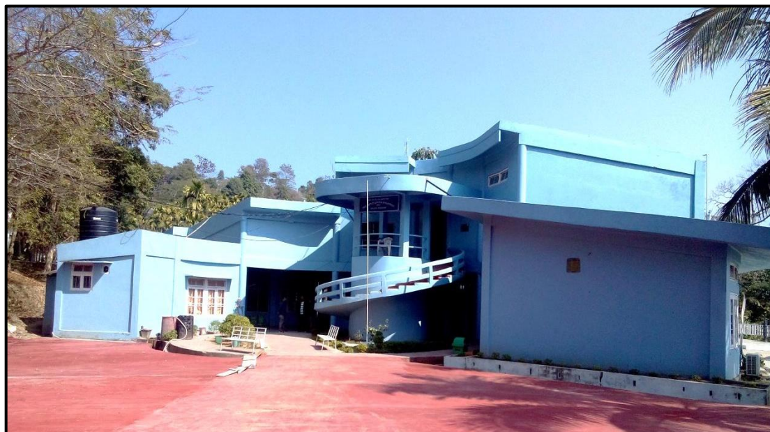
Administrative Building, ETC, Kolasib
