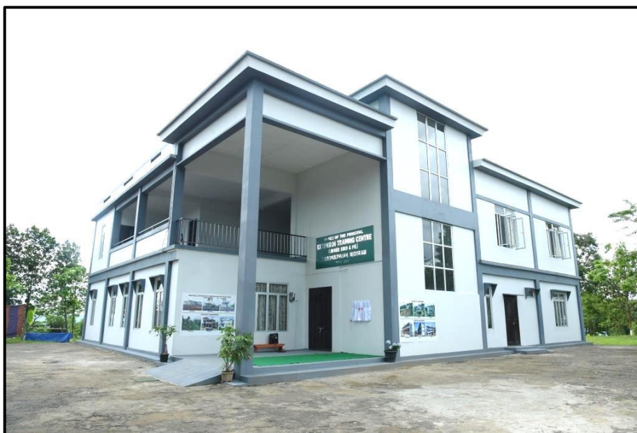
Administrative Building, ETC, Thingsulthliah
