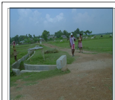
Fig.39: CONSTRUCTION OF PUCCA DRAIN
