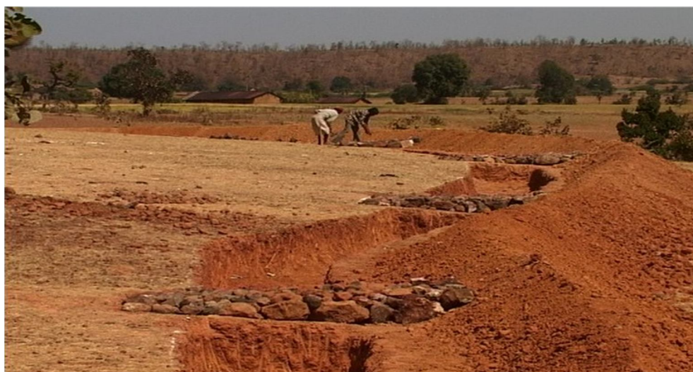
Figure 9: Earthen contour bund.
