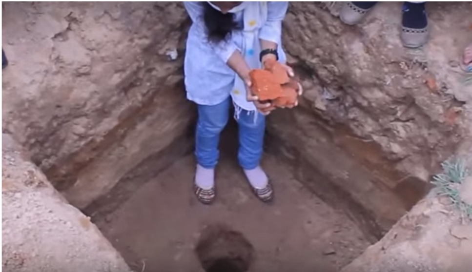
Figure 17: Recharge pit & Soak pit preparation.
