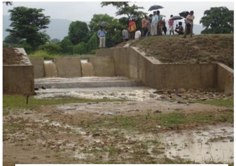
Fig.42. Down Stream of the Diversion Weir
