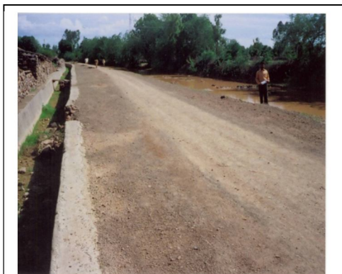
Fig 38: CONSTRUCTION OF PUCCA DRAIN
